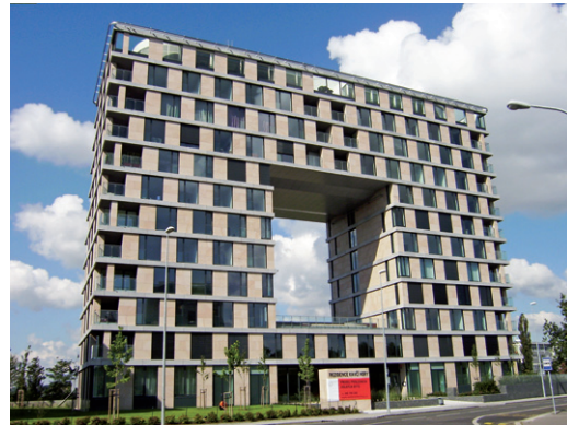
Residence Kavčí hory, Praha 4
